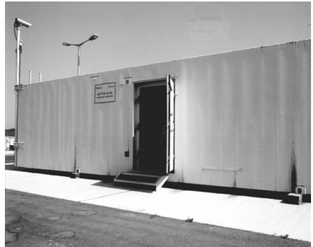
Command Electronics Shelter
